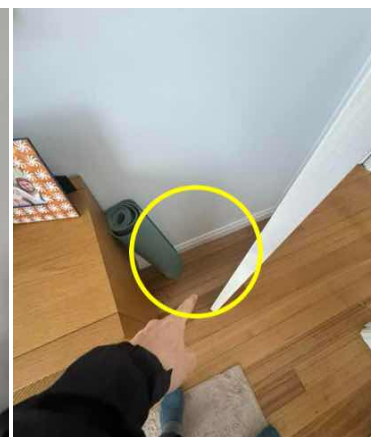
Door stops missing
